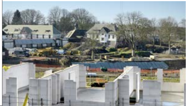
BELLA VITA Waterloo FCM Architects - Baudouin Courtens & Associés
